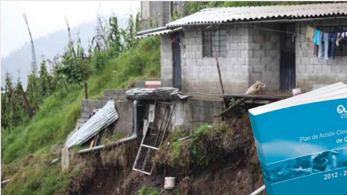
Inadequate housing on a steep slope in Quito. © Agencia Pública de Noticias de Quito
