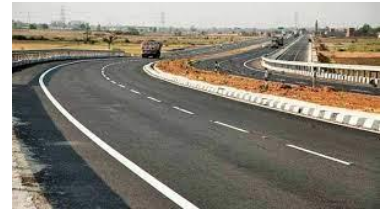
Glopram helps evaluate costs and benefits of PPP projects. Above: highway in India
